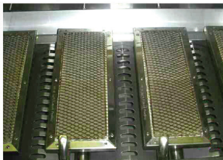
Multiple Sear Zone burners installed
